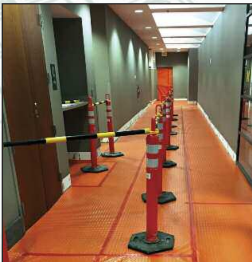
Guide foot traffic with safety delineators post and bars
